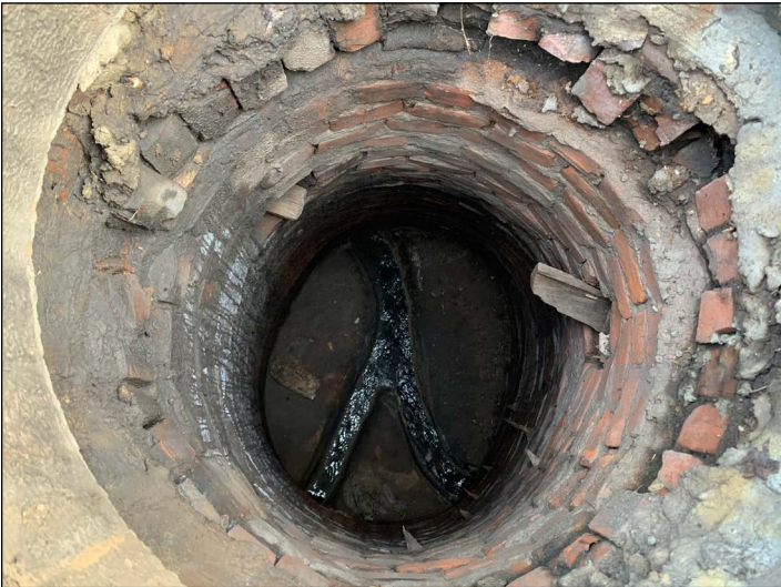
Figure 6: Manhole on West Plaza, with loose bricks, broken wood component, and sediment accumulation.
