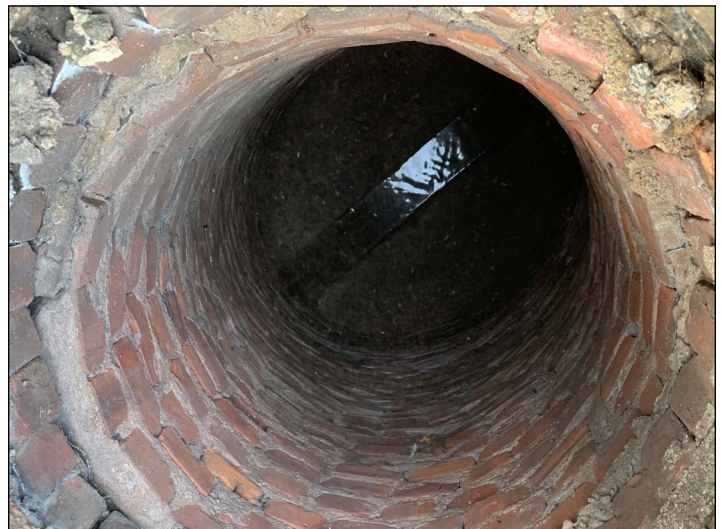
Figure 9: Manhole on West Plaza, with loose bricks and missing mortar.
