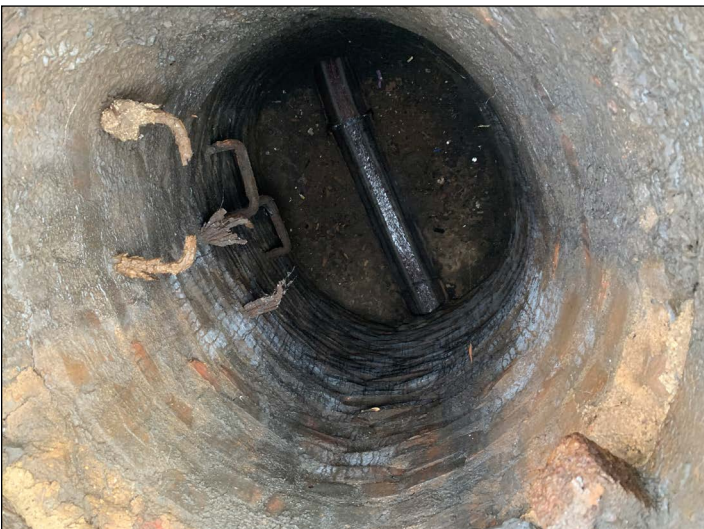
Figure 10: Manhole on Vreeland Avenue, with broken ladder rungs.
