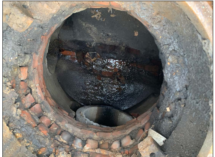
Figure 7: Manhole on West Plaza, with loose bricks, sediment accumulation, and asphalt previously used for repairs.
