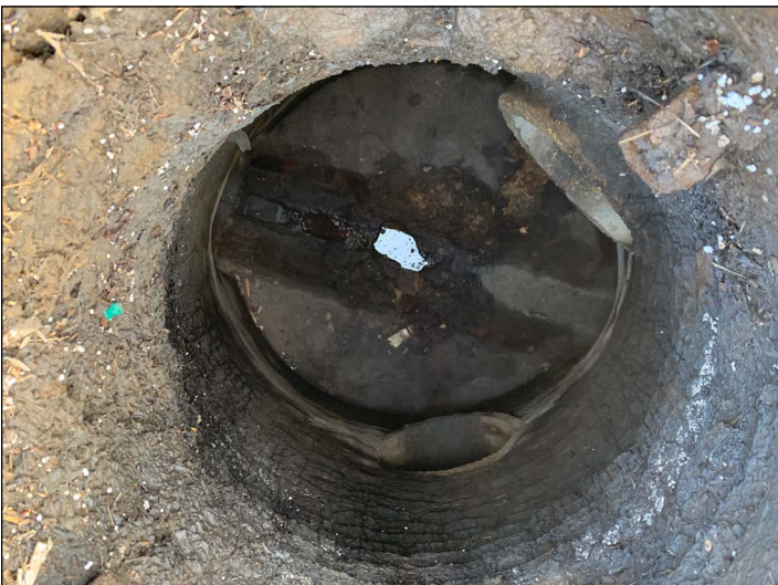
Figure 8: Manhole on Franklin Avenue, with sediment accumulation, and asphalt previously used for repairs.
